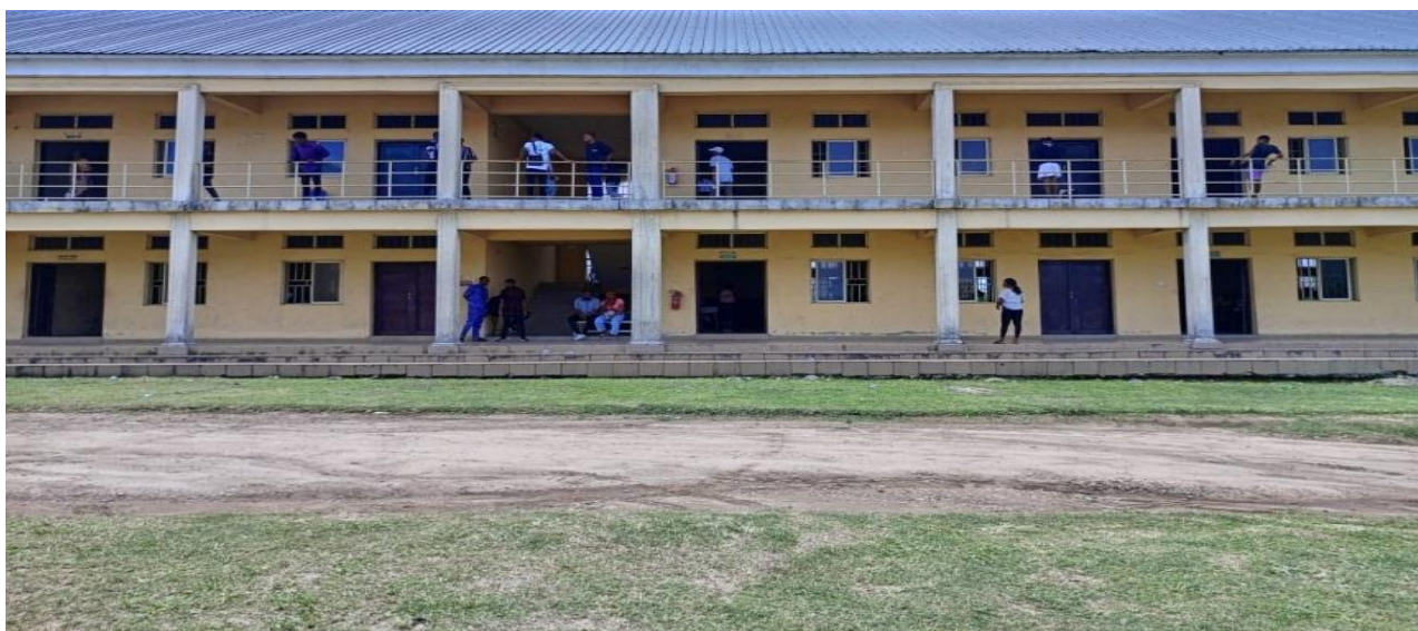
Fig. 2: A Disability-unfriendly Storey-building Classroom Block for Social Sciences & Postgraduate Students at Obio Akpa Campus. Source: Authors' Fieldwork, 2023
