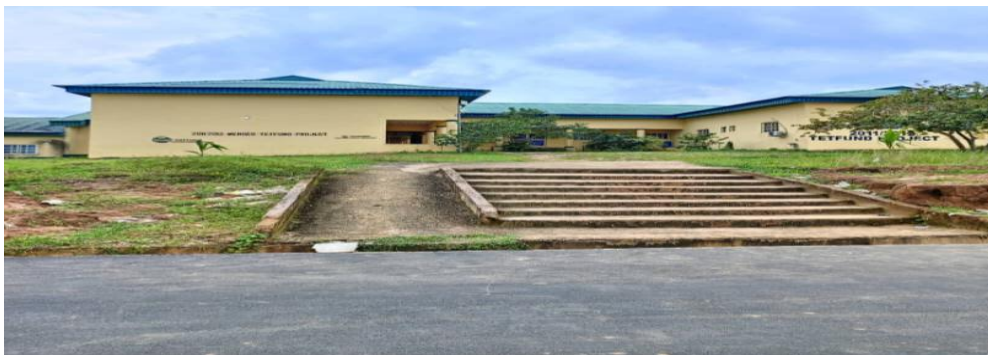
Fig. 4: Recommended for provision of slab to link the road with the ramp for a seamless access by wheelchair users on the campus to the Faculty building. Source: Authors' Fieldwork, 2023
