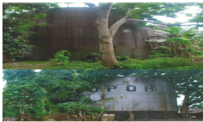
B.O.P. Tanks for Oil Storage and Reservoir at Abonnema Source: Field work 2013. Photograph by Mr. Uduak Akpan 12 September, 2013.
