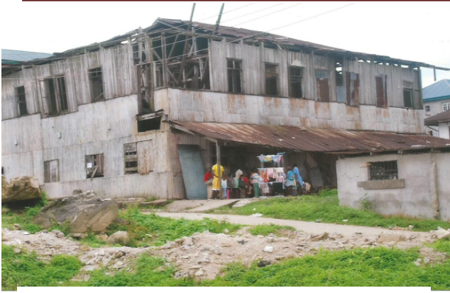
African Trading Company's Warehouse at Abonnema Photo credit: Mr. Uduak Akpan (12 September, 2013).
